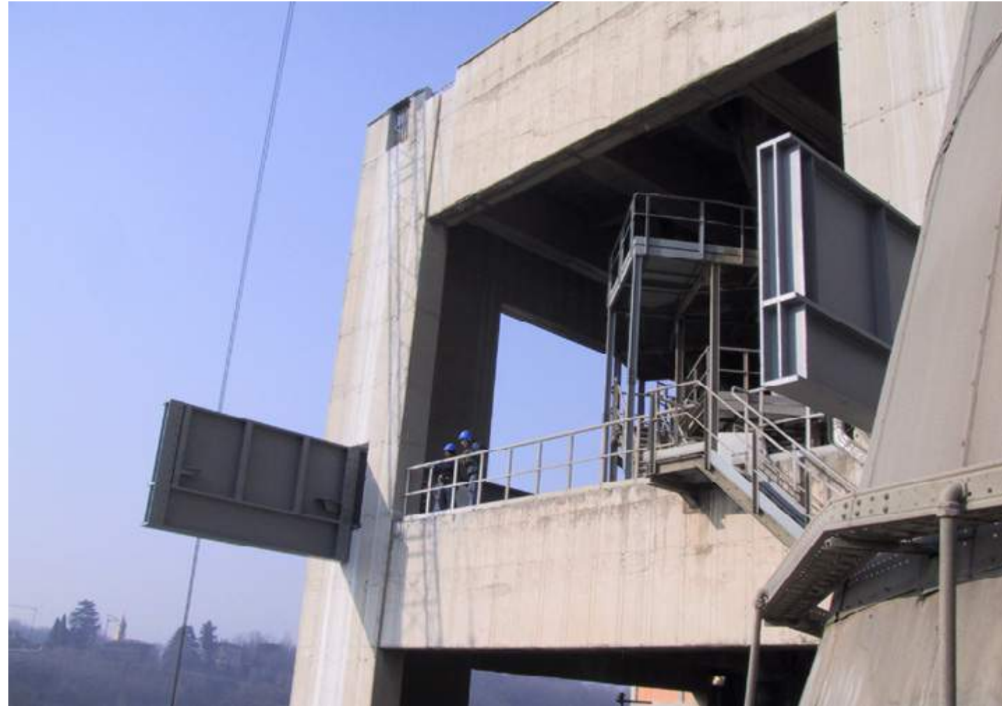
STRUCTURAL REINFORCEMENT OF A PRE-HEATER TOWER
